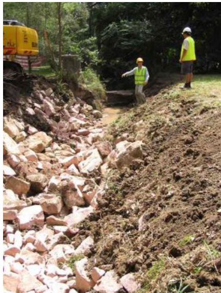
Above and below: Examples of the structural works installed to reduce erosion
