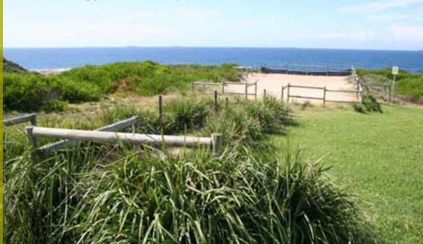
March 2008: Crabs Beach Landcare were involved in the construction of a whale watching platform and improved visitor access.
