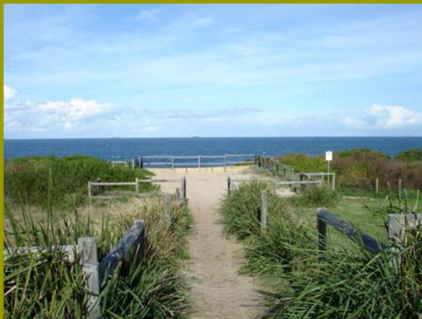
May 2010: Whale watch platform with the addition of timber boards at the base of the fence to stop erosion.
